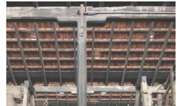
Figure 73: Wooden trusses are used for the whole roofing system [Source: Taken By Author]
