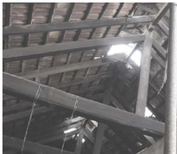
Figure 134: Image of king post truss roof frame [Source: Taken By Author]
