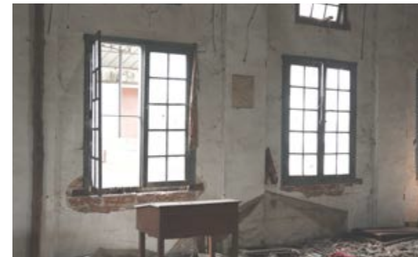
Figure 71: Brick and lime mortar is used for the basic wall construction [Source: Taken By Author]
