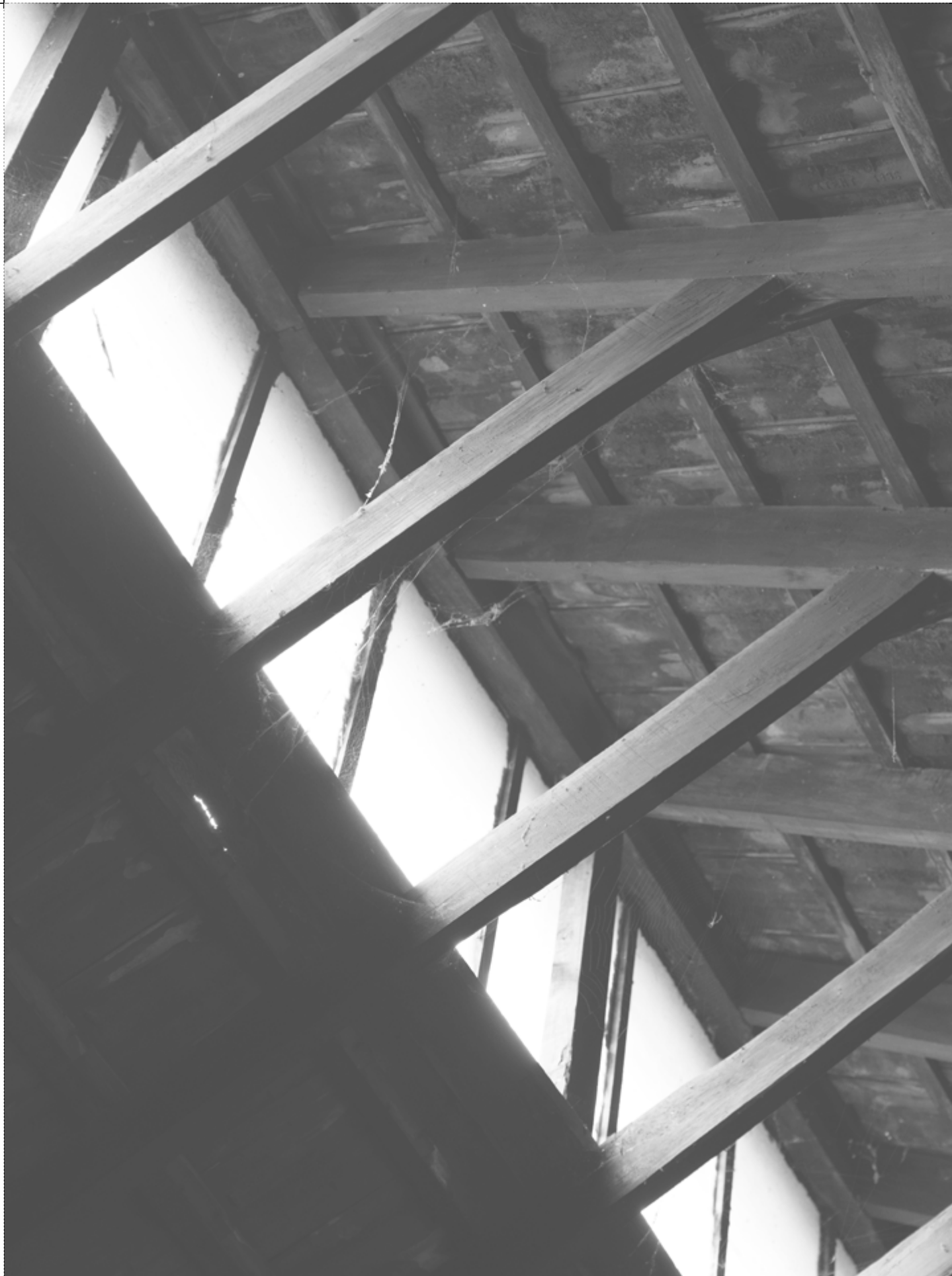
Figure 91: Image of the clearstorey glass windows enveloped with the sawtooth roof [Source: Taken By Author]
